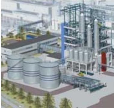
The plant started production in November 2002, just 13 months after work began, and at full capacity will achieve 150,000 tons a year. Over 300 intelligent field devices were supplied by Emerson, approved intrinsically safe for use in a hazardous area, according to the FISCO concept. Instrumentation included Rosemount temperature and pressure transmitters, and pH meters and toroidal conductivity measurement systems from Rosemount Analytical.
