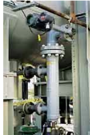
Field-mounted DeltaV controllers and I/O modules for the naphtha stabilizer, top row also serving the tank farm and pipeline and Crude Unit No. 1
