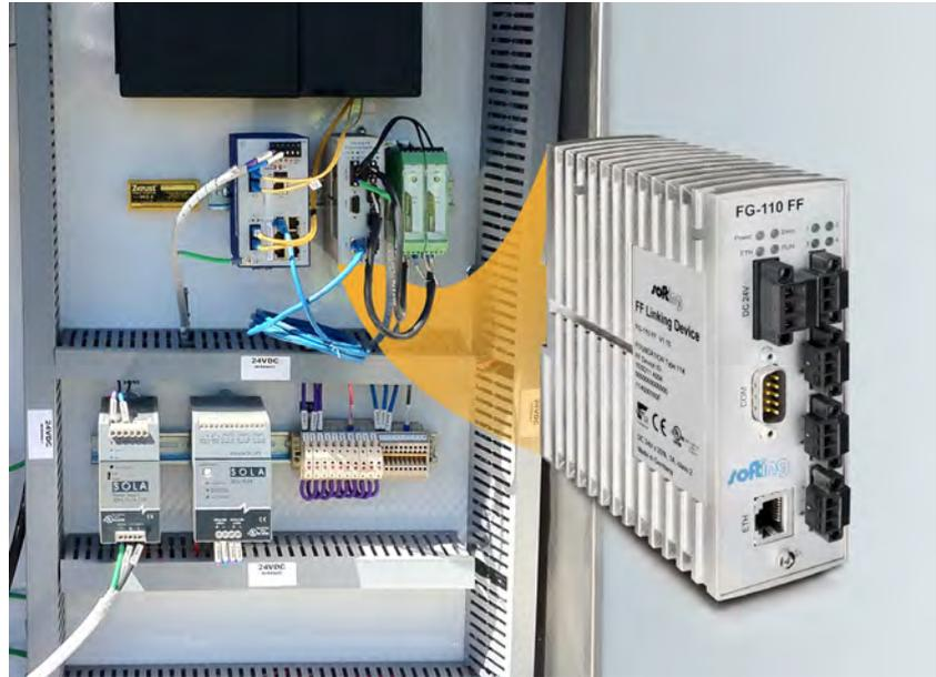
Figure 3: Remote cabinets located at the individual wells house the FG-110 FF gateway.
